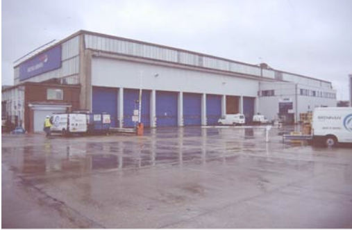
Gatwick Hangar 1 (external) © Ian Anderson
