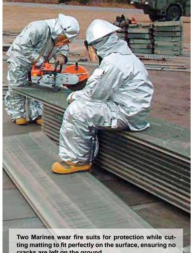
**Two Marines wear fire suits for protection while cutting matting to fit perfectly on the surface, ensuring no cracks are left on the ground.**
