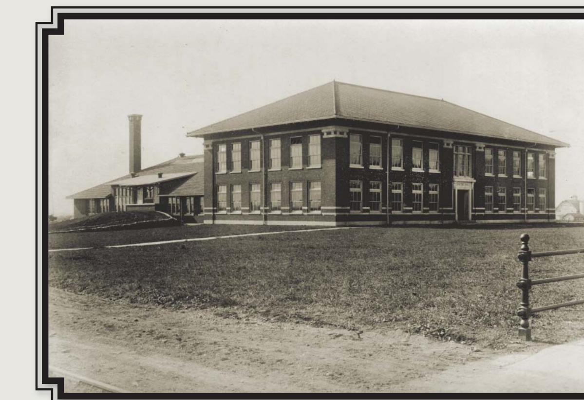
Smith Hall and adjacent creamery, completed in 1914
