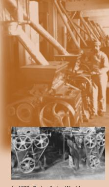
In 1879, Cadwallader Washburn installed a new steel roller milling system in his C mill on an experimental basis to demonstrate the value of rollers compared to millstones. It was the first complete automatic roller mill in the world.
