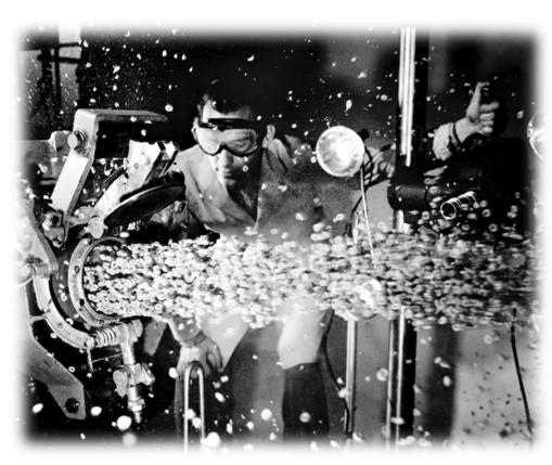
The puffing gun, developed in the late 1930s by General Mills engineer and chemist Thomas R. James, allowed the company to expand or "puff" pellets into different cereal shapes. It was the crucial technology component in the development of Kix cereal in 1937, and would be used to create Cheerioats in 1941.
