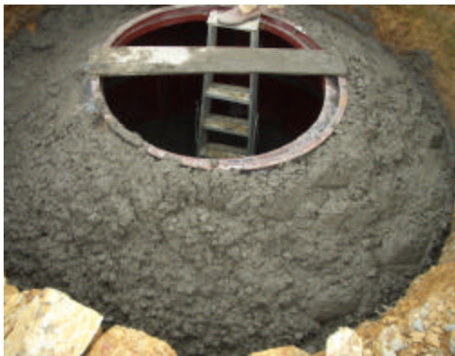
Construction for Lower Part
