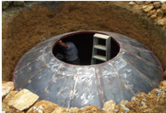
Fitting Lower Mould
