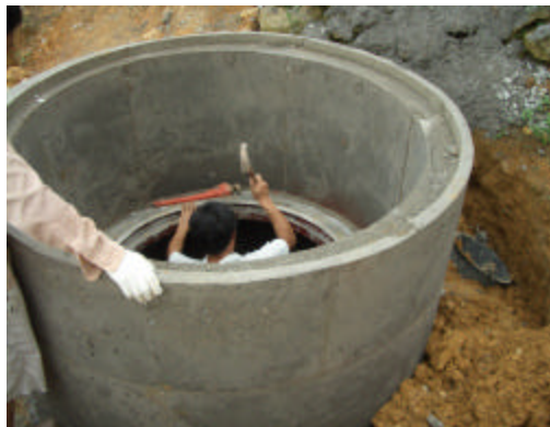
Final Construction of Upper Neck
