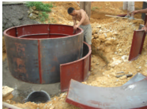
Fitting Upper Mould
