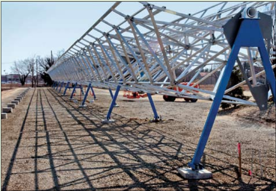
Lenny Johnson, maintenance mechanic, at left, and Chris Myers, vice president of the solar energy program at MS2 in Moorestown, N.J., examine the frame for the solar test bed under construction, called Solar System Test and Engineering Site Array. The photo below shows the frame, which will hold the large mirrors.
