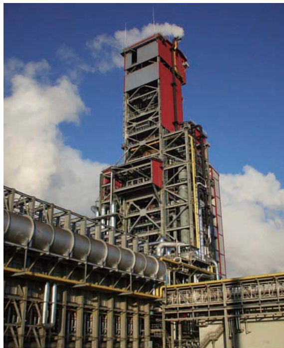
A direct reduction plant using the MIDREX® Process for the Lebedinsky Mining and Processing Integrated Works in Russia
