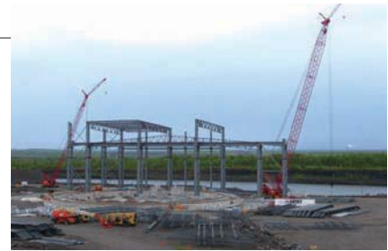
Construction of the first commercial ITmk3 ® plant in Minnesota, USA
