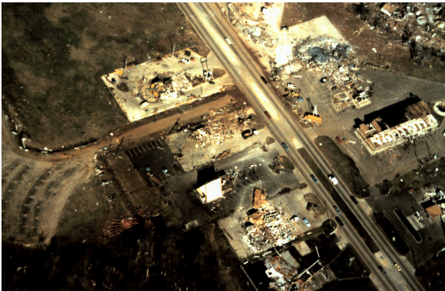
Airline Drive Area. The pointed roof of the Whataburger is left untouched. Structures on both sides were smashed by estimated upper F3 to lower F4 winds. Starbucks is now in the approximate location of Whatburger. (Photo courtesy of Ernest Ethridge)
