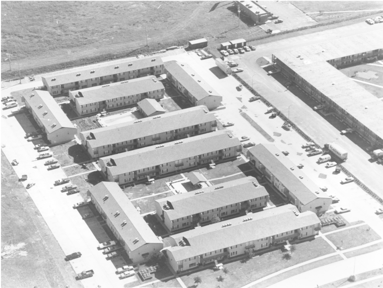
The Port au Prince Apartments in Bossier City almost 1 year after the Bossier City tornado. (Courtesy of LSUS Archives – Noel Memorial Library)
