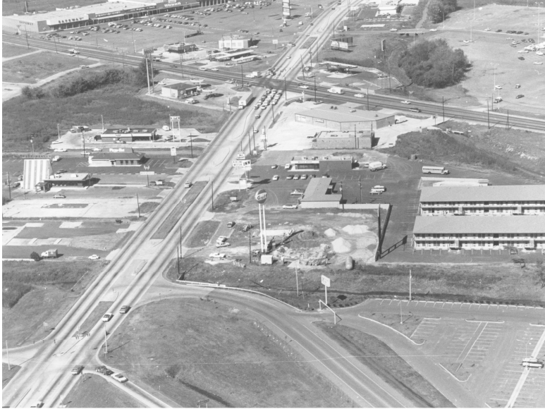
Looking north on Airline Drive almost 1 year after the Bossier City tornado. The location of the Pizza Hut has not changed and is seen on the left adjacent to Whataburger. (Courtesy of LSUS Archives – Noel Memorial Library)
