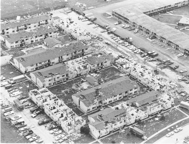
Damage to the Port au Prince Apartments in Bossier City. (Courtesy of LSUS Archives – Noel Memorial Library)
