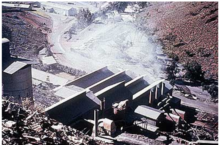
Airborne asbestos dust visible outside the mill
