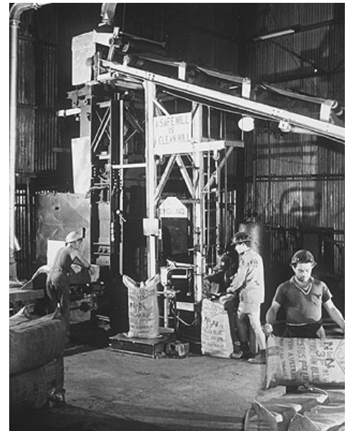
New Bagging Plant
