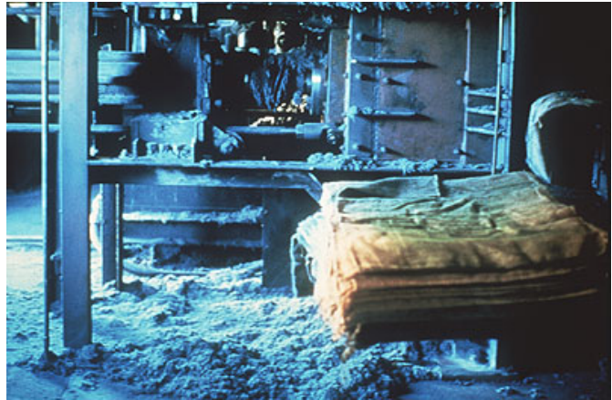
Asbestos bagging area at the mill
