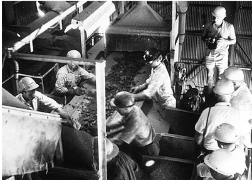
'Pickers' remove larger pieces of rock from the moving conveyor belt
