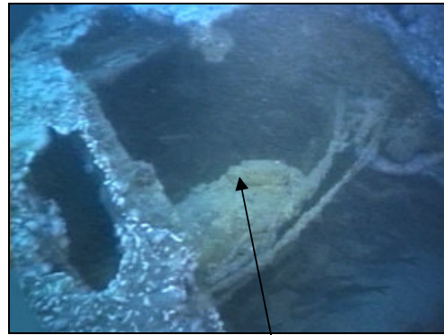
Figure 42: Heater Unit in situ.
