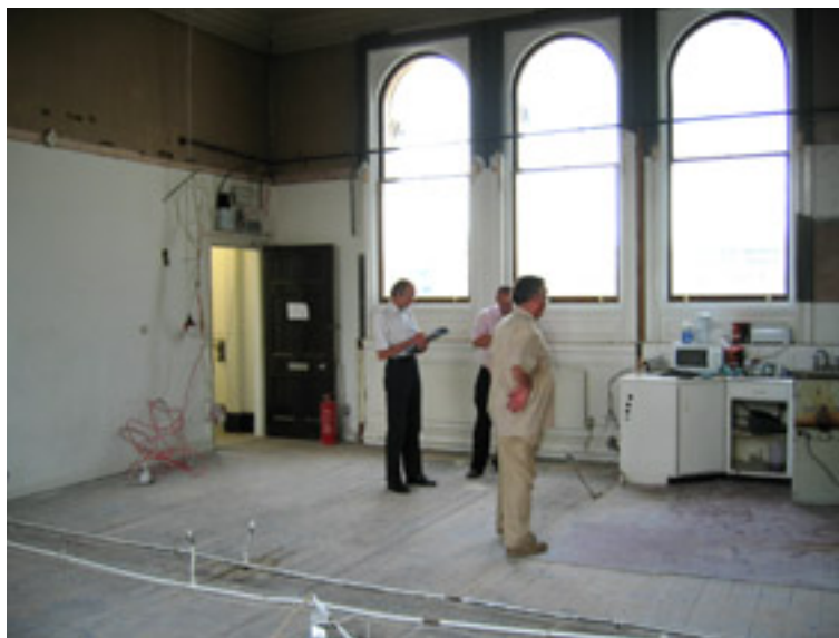
The Treasurer, Prof. Gren Lucas, and the Executive Secretary Adrian Thomas (left) inspecting one of the Tower Rooms which is due for restoration.
