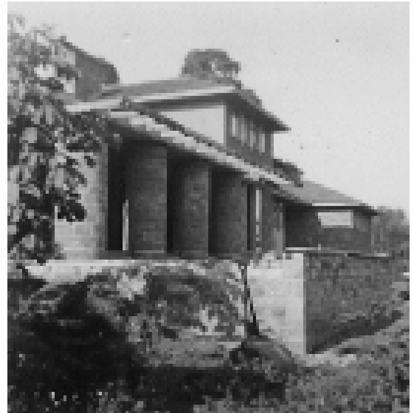
7.7 The pillars were beautiful modern examples of the ancient art of stonemasonry
