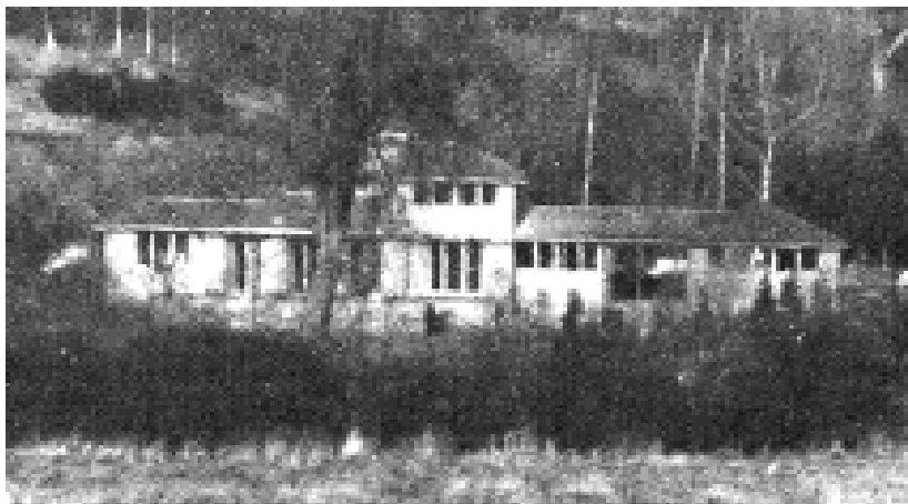
7.6 Robinswood nearing completion.
