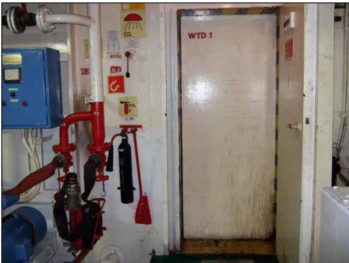
Photograph of watertight door No.1 (closed) - view from changing room
