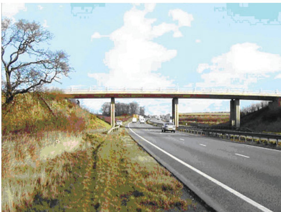
Plate 2-2: Typical Rural All Purpose Dual Carriageway Cross-section
