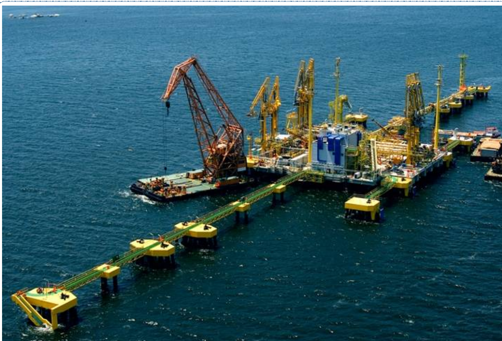
Terminal Overview: Construction and Assembly (C&A) Completion – 01/22/09
