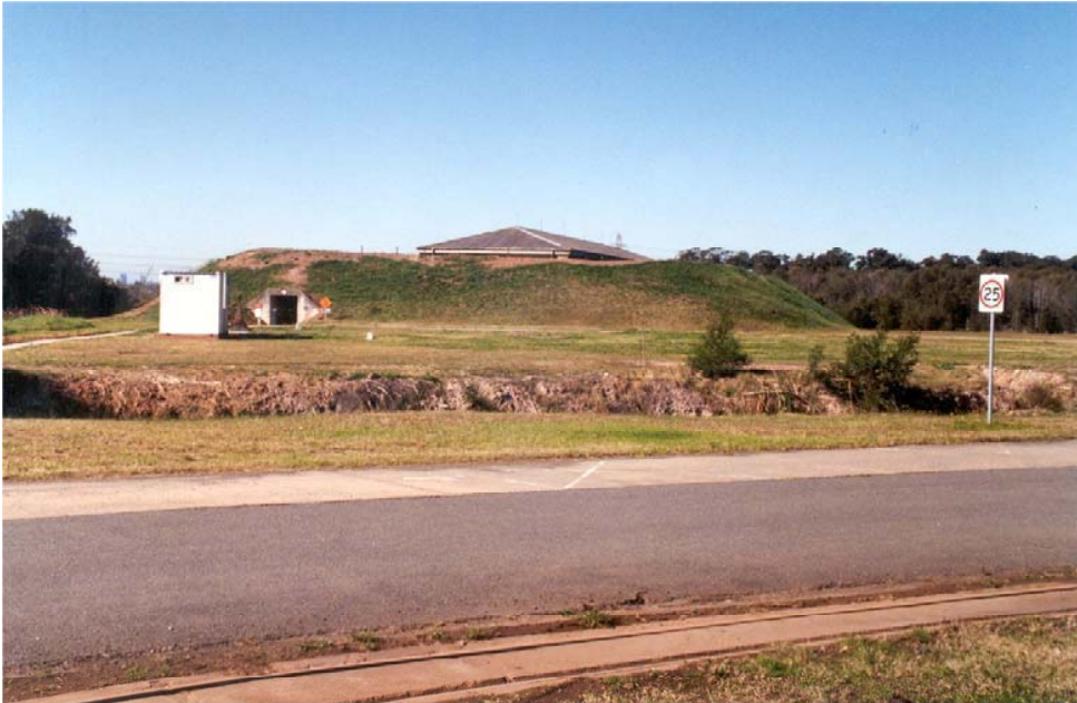
Figure 3.33. Large RAN Explosives Storehouse (18) protected by earth traverse Schwager Brooks and Partners 1996
