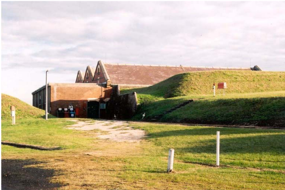
Figure 3.5. Original Gun Powder Magazine (20) with protective earthworks
