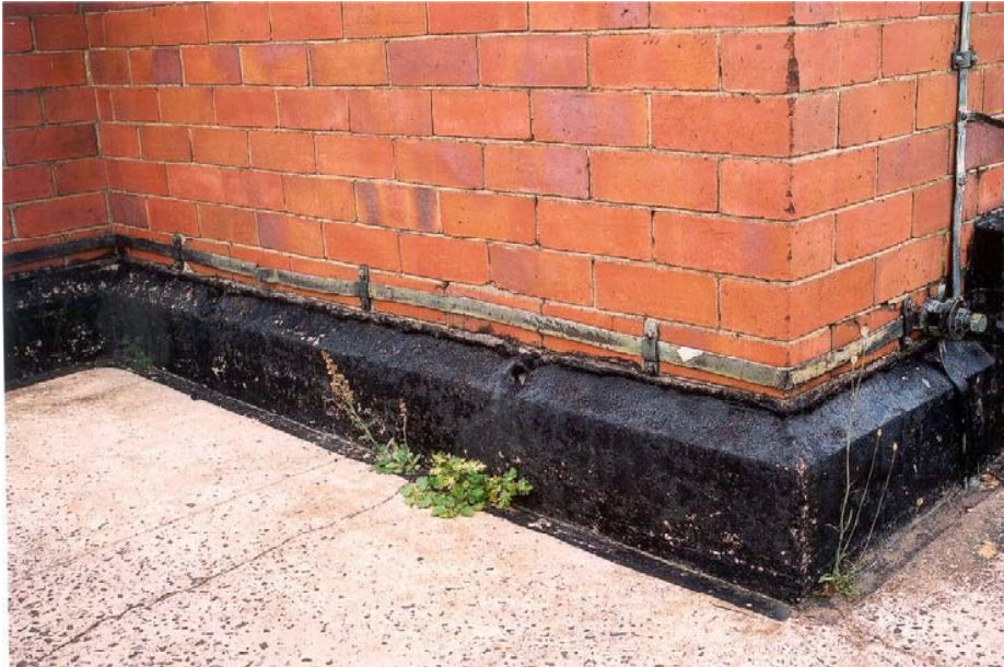
Figure 3.26. All external elements of workshops and storehouses are fitted with earthing conductors. Schwager Brooks and Partners, 1996
