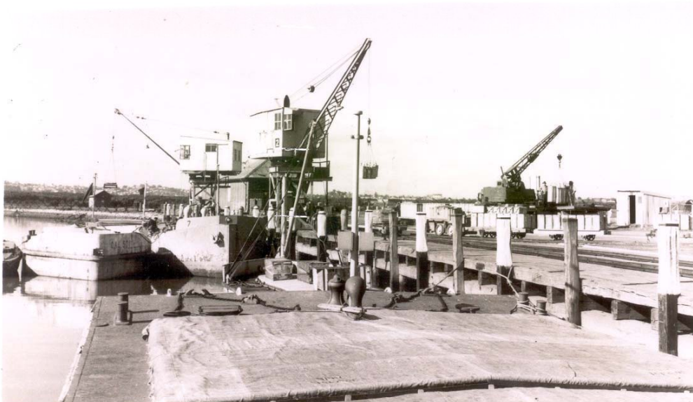
Figure 3.24. Cranes, lighters and rail transport on the wharf, 1950s Schwager Brooks and Partners 1996
