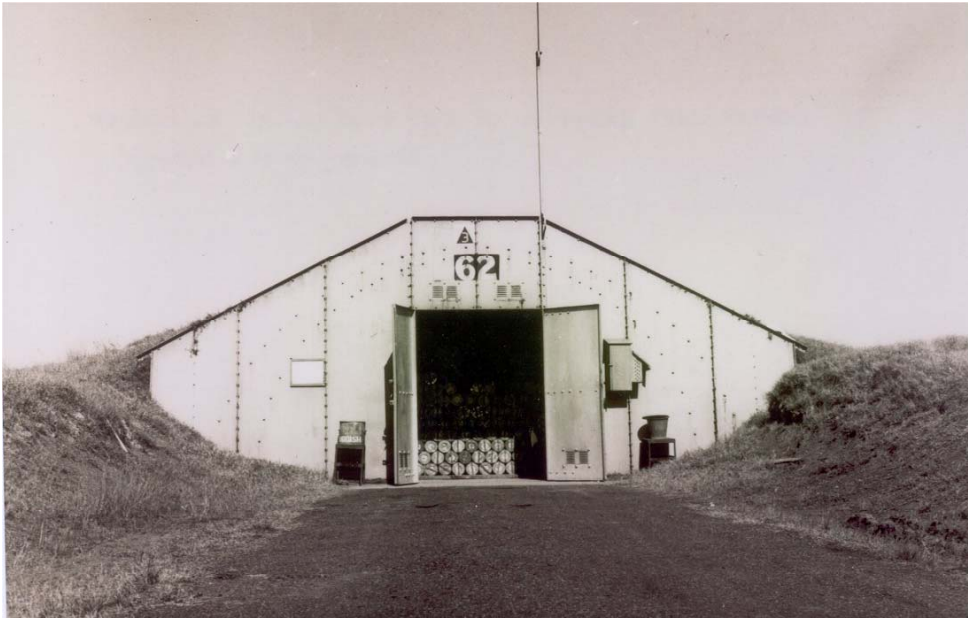
Figure 3.16. Steel Armco style US Navy Explosives Storehouse now demolished, 1950s Schwager Brooks, and Partners 1996
