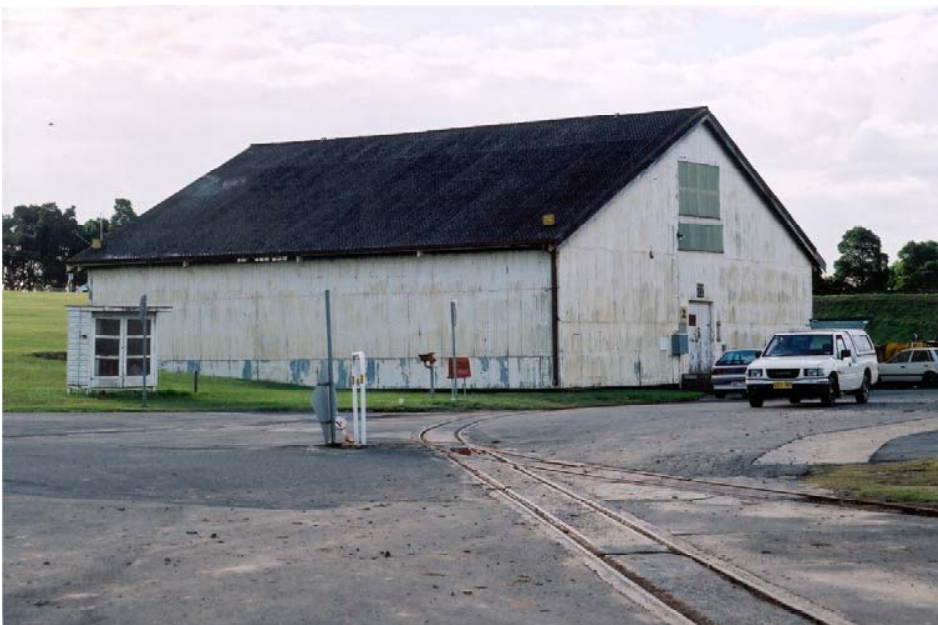
Figure 3.10. Non-explosives store at centre of site (22)
