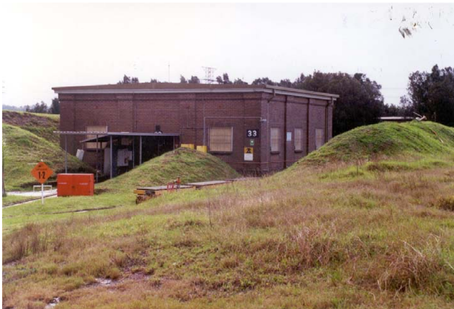
Figure 3.32. RAN pre-WWII explosives storehouse (33)
