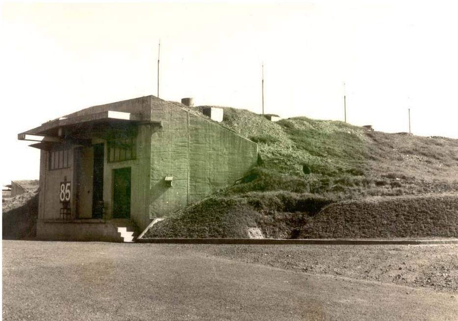
Figure 3.35. Former single concrete box style underground explosives storehouse (85) now demolished. Schwager Brooks and Partners, 1996
