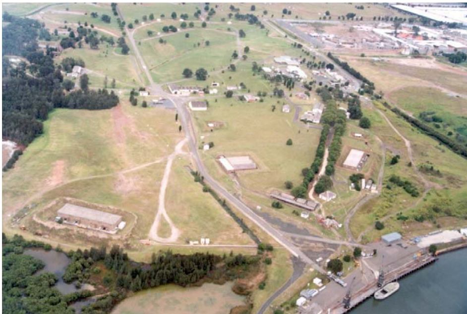
Figure 1.7 Aerial Photo from the north, prior to Sydney 2000 Olympic and Paralympic Games related works, 1996 Schwager Brooks and Partners
