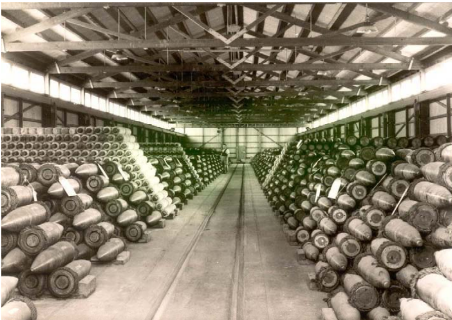
Figure 3.15. Interior of Building 26, 1950s Schwager Brooks, and Partners 1996
