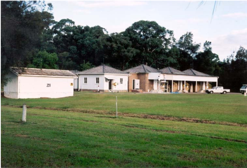
Figure 3.9. A row of explosives workshops (130-134) with woodland backdrop
