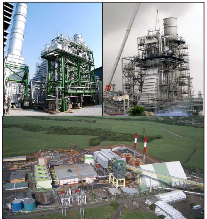
2007 WAS A VERY SUCCESSFUL YEAR FOR OUR CURRENT CONTRACTS TOP LEFT - NPC III COGENERATION THAILAND; TOP RIGHT - THAI OIL HRSG BOTTOM - SAVANNAH COAL & BAGASSE FIRED POWER PLANT, MAURITIUS
