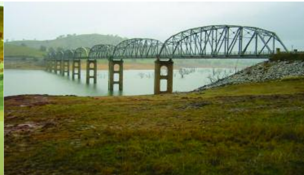
Above: Bethanga Bridge
