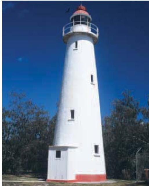
The historical significance of Lady Elliot Island Lighthouse has been recognised through its inclusion on the Commonwealth Heritage List.
