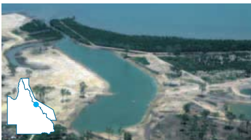
The natural environment and drainage patterns are substantially changed in most coastal habitats altered for urban expansion such as this development near Cardwell.
