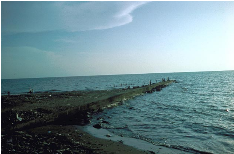
Figure 5.8 Sewage and stormwater outlet for the 'Old City', Al Hudaydah.
