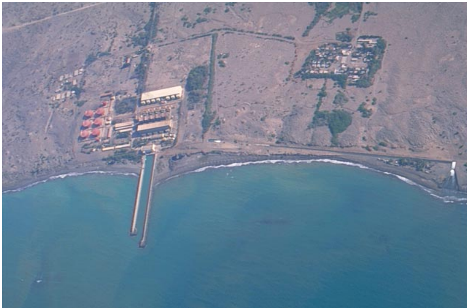
Figure 5.3 Power station north of Al Hudaydah.
