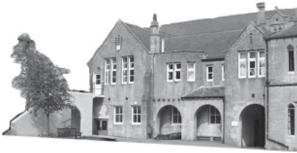
The 1891 wing which houses the current first floor KA Office
