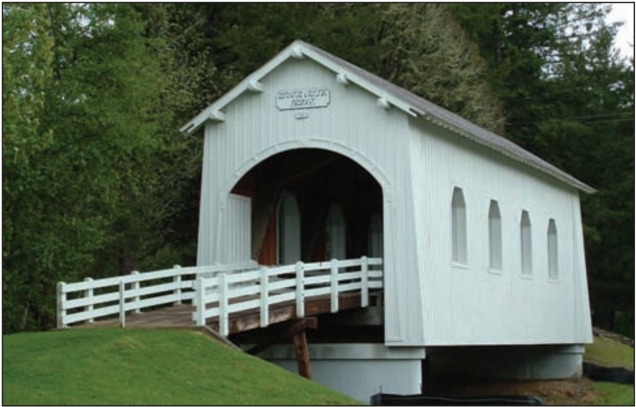
The historic Ritner Creek Bridge underwent a major restoration effort to bring it back to its grand self.
