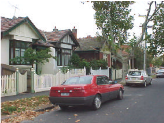
Figure 3 South side of Godfrey Avenue
