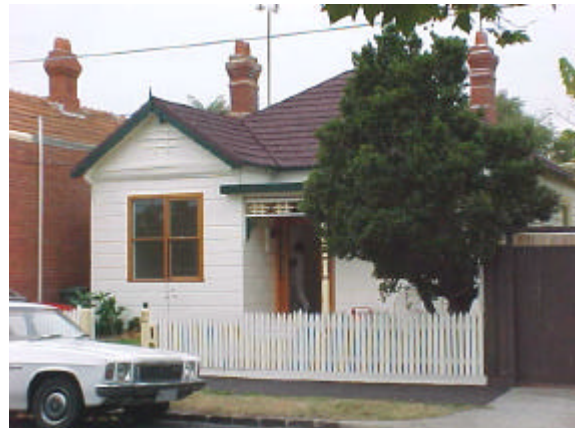
Figure 4 Weatherboard house at No 2
