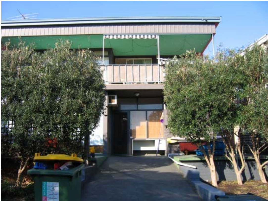
Example 2 - Level 0 entry into ancillary accommodation in Compound House 2.
