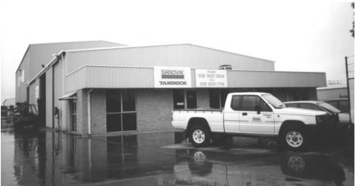
Sandvik Tamrock's Western Region Distribution Centre situated in Kalgoorlie.
