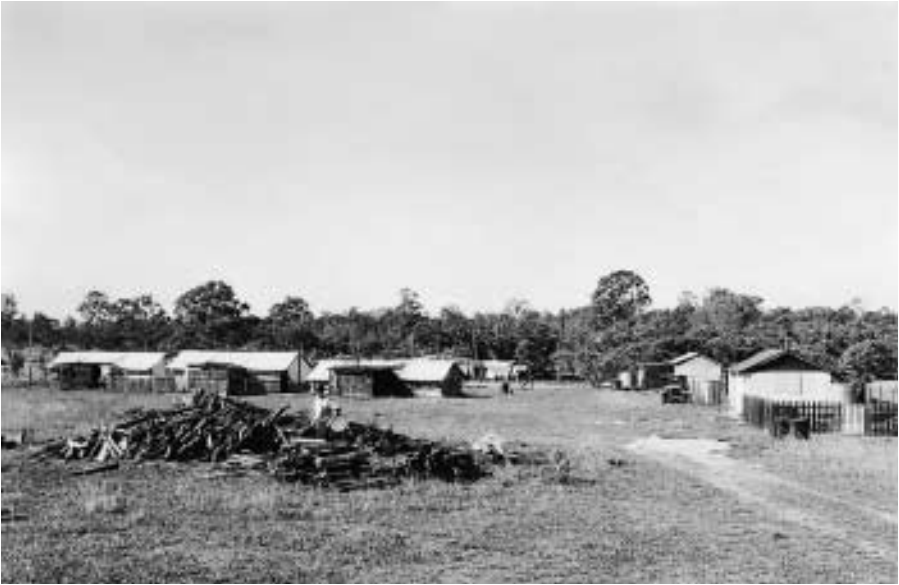
Typical survey camp, Caboolture, 1952. Surveying teams withstood trying conditions in order to expand Queensland's road network.
