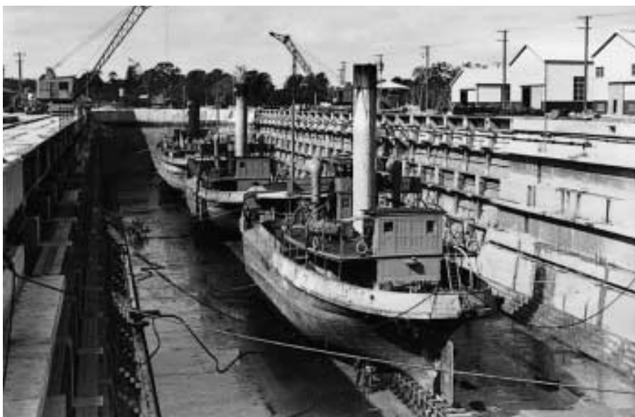
The Cairncross Drydock – one of the key defence projects undertaken during the war years.
