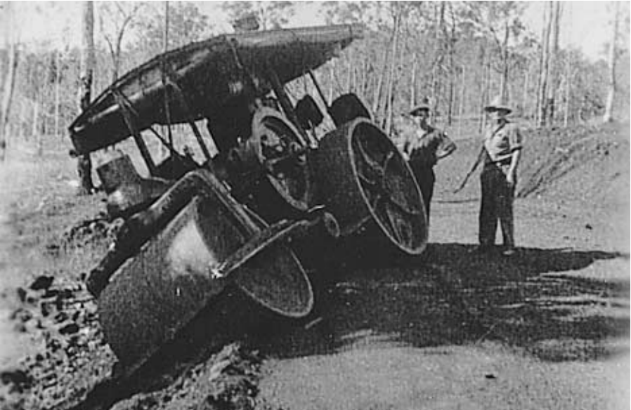
Perhaps it was only minor assistance at first, but the business of building roads was made a little easier with mechanical help provided by the steamroller.
