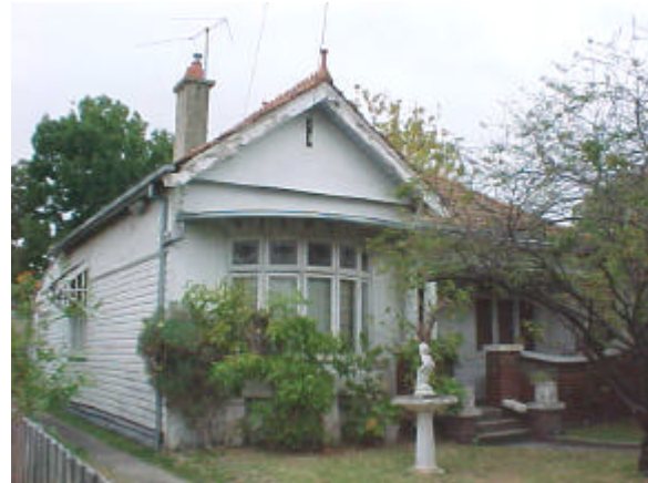
Figure 4 Weatherboard house at No 6
