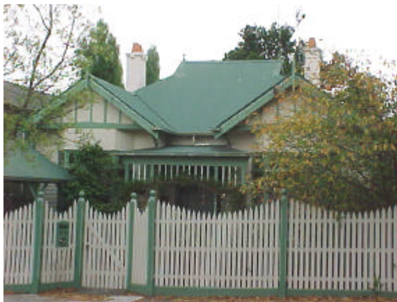
Figure 5 Weatherboard house at No 27
