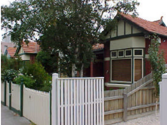
Figure 1 Row of houses, 1-7 Kalymna Grove
