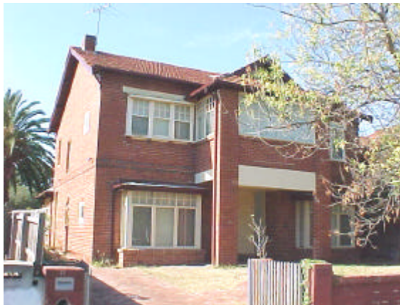
Figure 4 Wittonia Flats at No 27 (c.1922)
