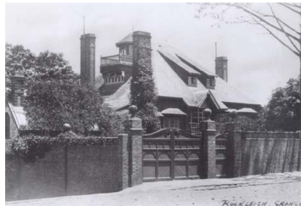
Rockleigh Grange after the extensive alterations and extensions, c.1905. Photograph by Harold Cazneaux (North Sydney Heritage Centre, PF 2055)
