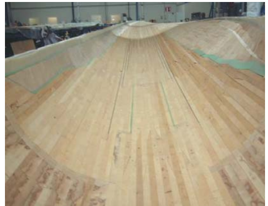
Above: Dry materials layed in the mould ready to be bagged.
