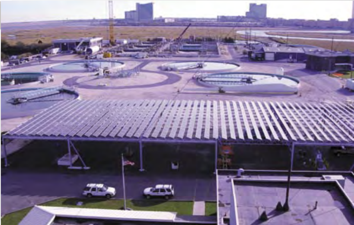
The Solar Canopy over the wastewater treatment facility parking lot soaks up the sun's rays and protects fleet vehicles from the elements.
