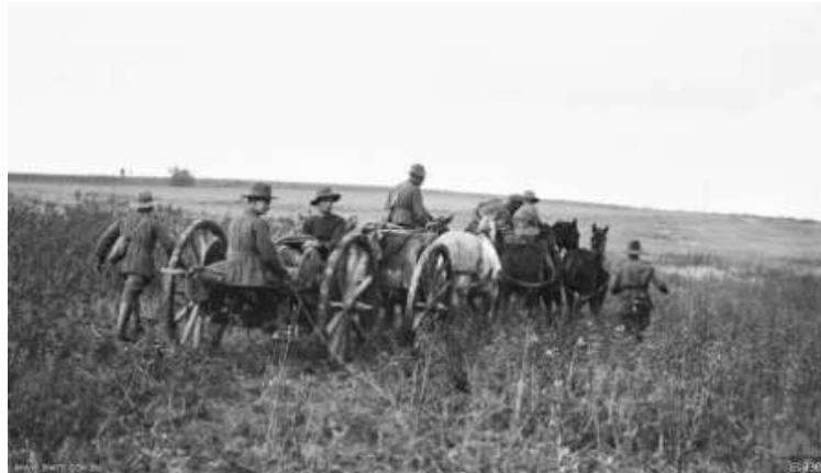
A cable section of the 3rd Divisional Signal Company laying a telephone cable near Ronssoy, when the 3rd Division assisted in retrieving the misfortune of the 27th American Division in the left sector over the canal tunnel against Bony and Le Catelet on the Main Hindenburg Line, 30 September, 1918. (Source: www.awm.gov.au )
