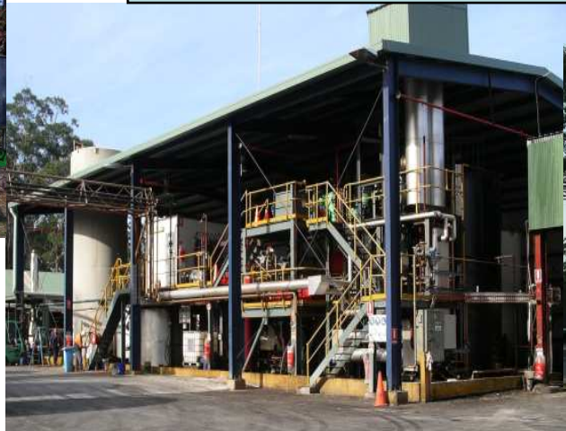
Initial Trial Mobile Batch Plant 2001 Design capacity 5000 l/day
