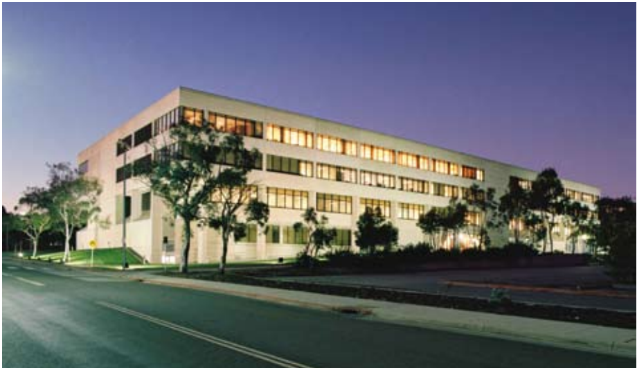
The ASIO-ONA Building
