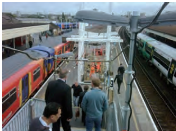
Clapham Junction Gap Station
