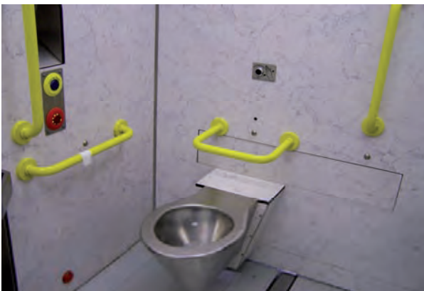
Liverpool South Parkway Disabled Facilities
