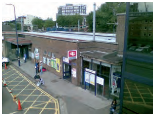
Luton Gap Station
