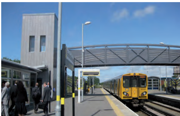
Bootle Oriel Road Access Lift
