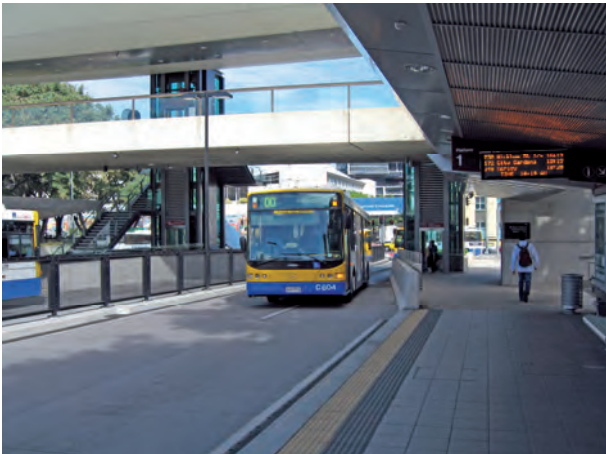
Brisbane Cultural Centre Interchange
