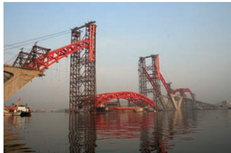
(b) Under construction
