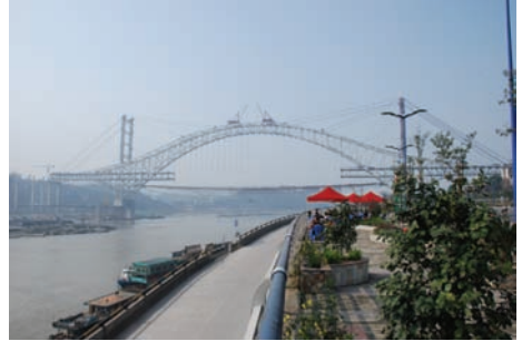
(b) under construction
