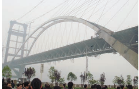
(b) Under construction
