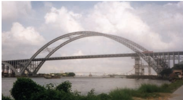
(c) Finished photo
