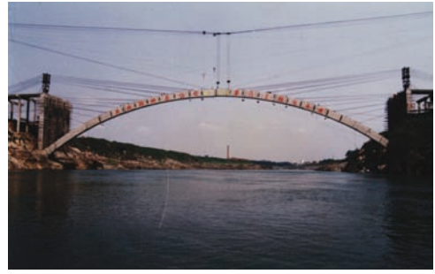
(b) Under construction
