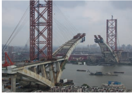
(b) Under construction
