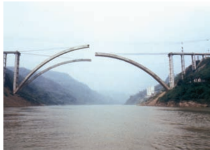
(b) Under construction
