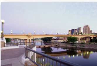
Wabasha Freedom Bridge -FIGG/TKDA
