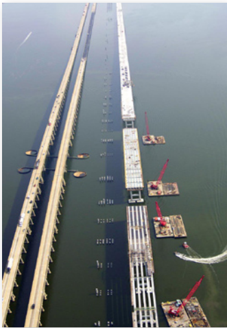
I-10 Bridges Pensacola - FLATIRON
