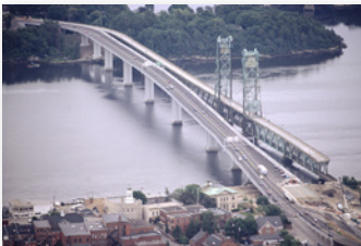
Sagadahoc Bridge - FLATIRON/FIGG
