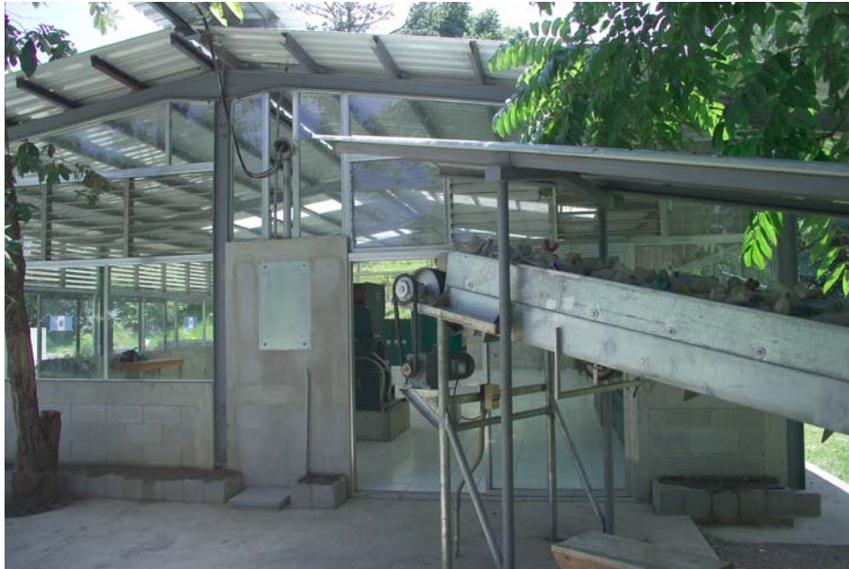
Figure 1: Plastic Recycling Plant
