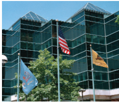
Downtown Milwaukee Campus 700 West State Street Milwaukee, WI
