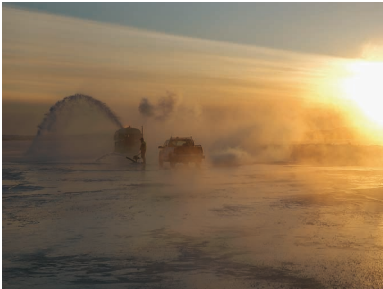
The winter road – the world’s longest ‘school zone’ – is constructed, operated, and monitored in a safe and environmentally responsible manner. To build thickness, work crews flood the ice surface.
