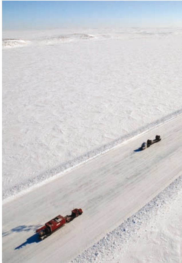
The winter road – the world’s longest ‘school zone’ – is constructed, operated, and monitored in a safe and environmentally responsible manner. To build thickness, work crews flood the ice surface.
