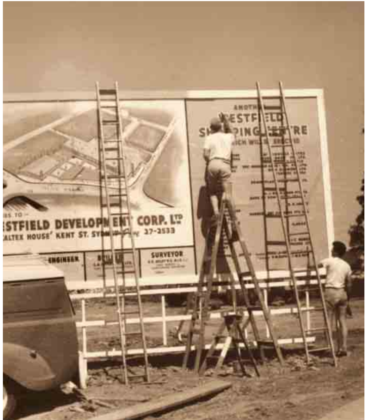
Putting up advertising billboards for the Hornsby centre prior to its construction.
