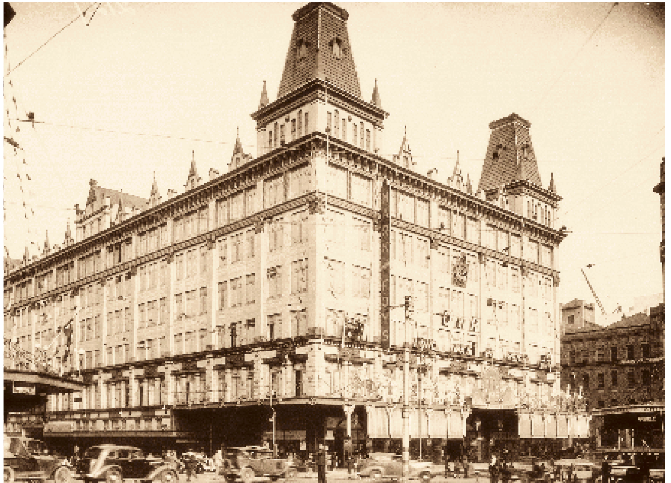
The grand and commanding Mark Foy's department store, set on a full city block, Sydney, 1939, ...
