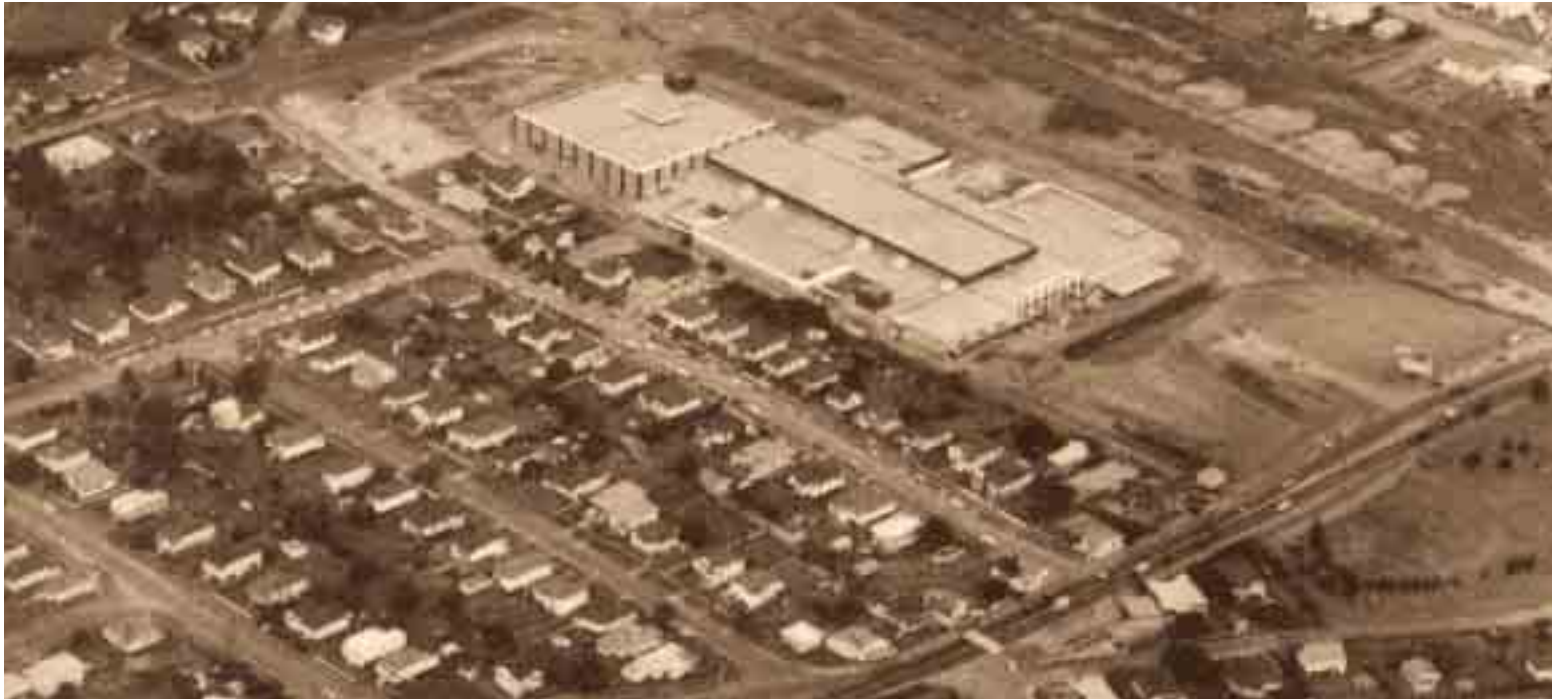
An aerial view of Toombul Shoppingtown under construction, showing the canal.
