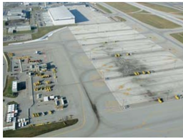
Central Deicing Facility
