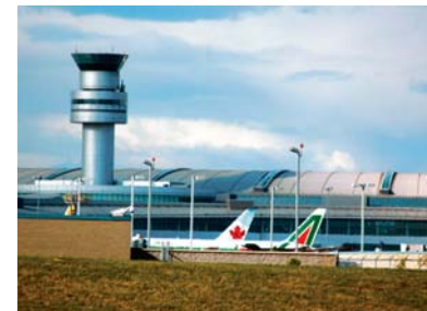
Terminal 1 Apron Control Tower
