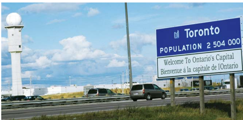
South ASDE Tower
