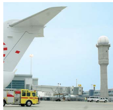
North ASDE Tower
