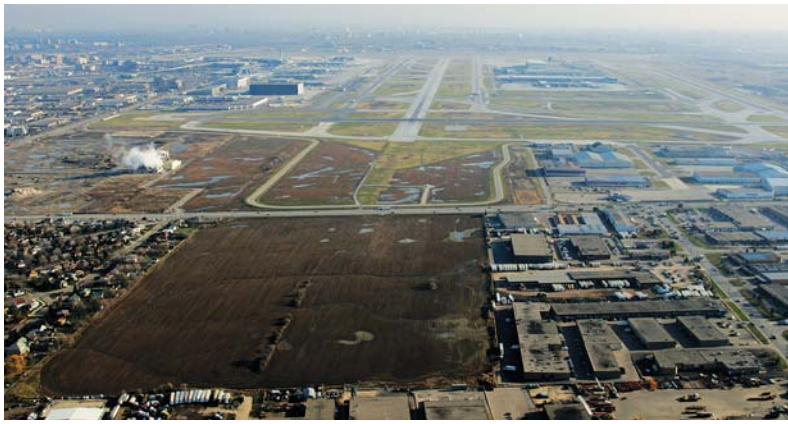
View of the Airside System from Airport North
