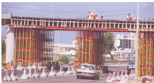
Repair of a war-damaged bridge
