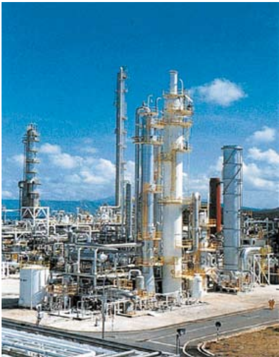
Figure 3.5 CO 2 capture plant in Malaysia using a 200 tonne d -1 KEPSCO/MHI chemical solvent process (Courtesy of Mitsubishi).
