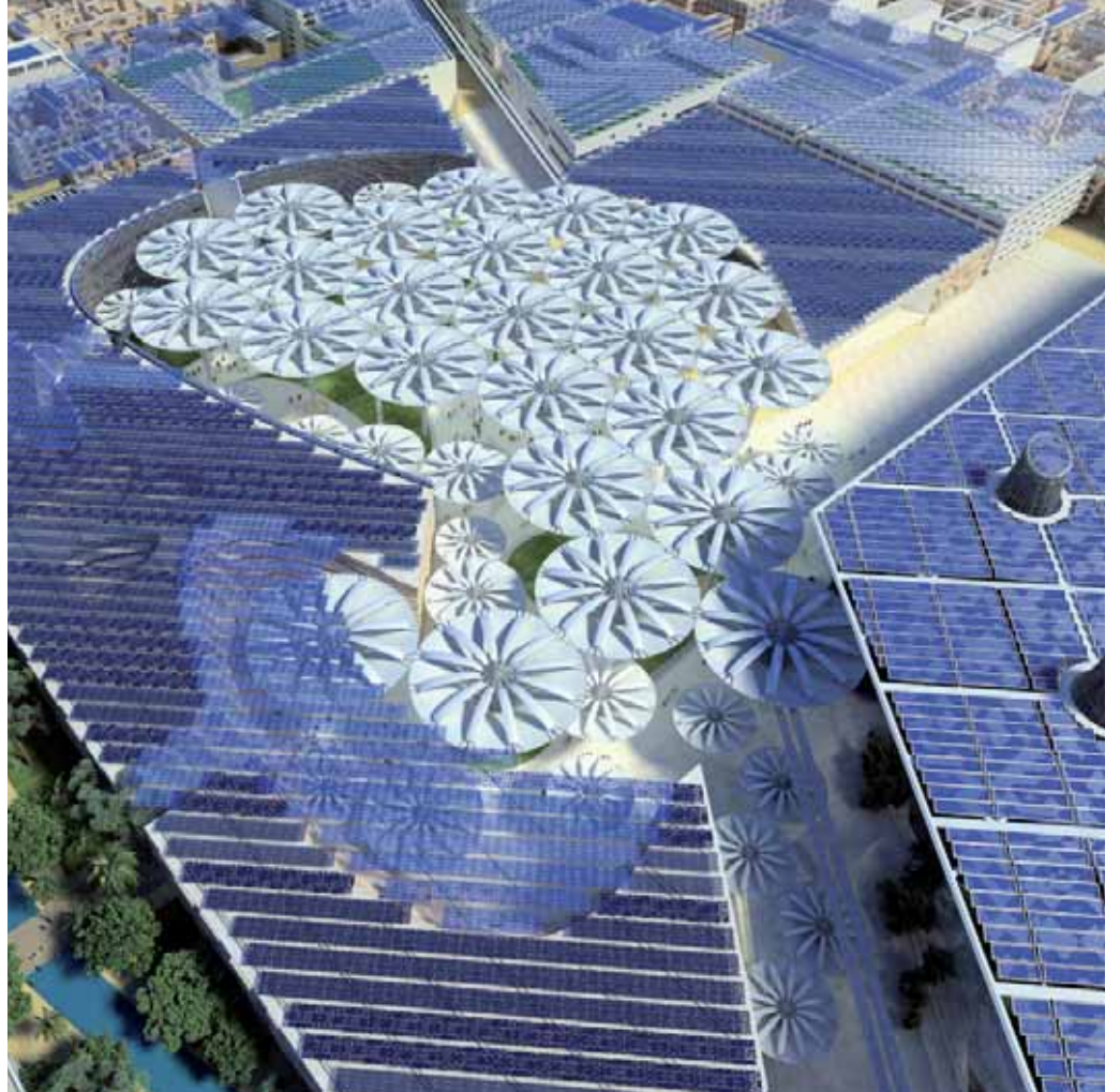
Masdar City's hotel and conference centre facility, designed by LAVA, will provide much of its own power from the photovoltaic arrays on its roof canopy.
