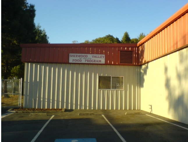
Figure A-21. SVFDPIR Headquarters Exterior
