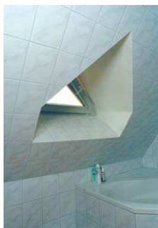
Tricky airtightness detail in the triangular dormer windows
