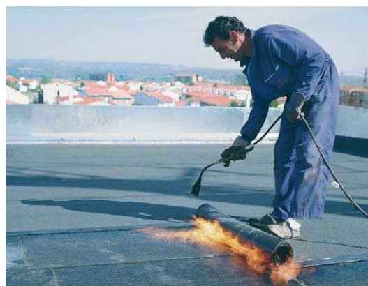
Renovation of the water-tight layer on a flat roof
