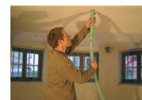
Insulation is blown into a T-beam ceiling
