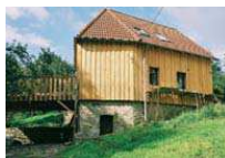
Outer insulation of a solid wall with a ventilated wooden facade over the entire area
