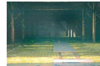
New insulation on top with an air- and vapour-tight foil underneath
