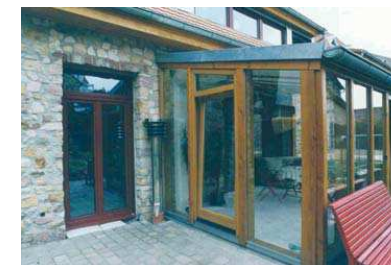
Fresh air routing of the geothermal heat exchanger via the terrace
