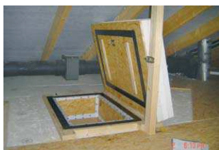
Insulated and airtight hatch leading to an unheated loft
