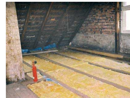
Loft ceiling opened from the top and insulated first between rafters
