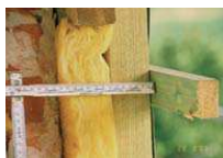
2 x 6 = 12 cm outer insulation of a solid wall with a ventilated wooden facade on the 1st floor
