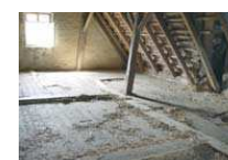
Wooden loft ceiling with beams visible from below
