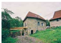
2 x 6 = 12 cm outer insulation of a solid wall with a ventilated wooden facade on the 1st floor
