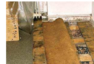
Wooden cellar ceiling, only partly opened for blow-in insulation
