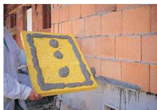
Correct application of the sealing compound
