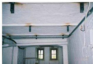
T-beam ceiling with freshly welded hangers for installing insulation from below
