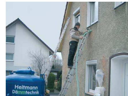
Blowing granular perlite insulation into a cavity wall
