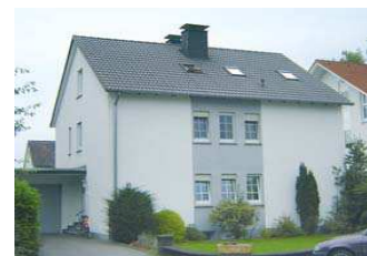
Multi-family house of the 1970s with added mechanical ventilation
