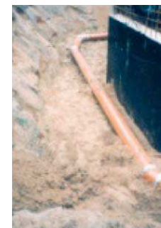
Geothermal heat exchanger with 200 mm sewage pipes laid around the cellar
