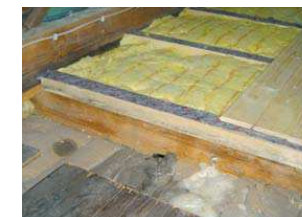
... and then between additional battens installed on top
