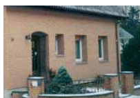
2 x 6 = 12 cm outer insulation of a solid wall with a clinker facade
