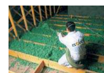
Wooden loft ceiling that must not be opened
