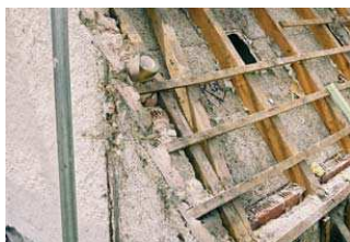
Plaster baseboard from outside with a recently opened roof
