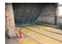
Ceiling opened and insulated from the top
