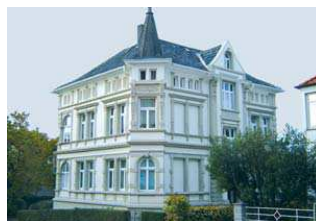
A candidate for insulation from inside: 5 cm will generate a 60 % heat loss reduction of the 36 cm brick walls.
