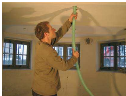
Wooden cellar ceiling: insulation is blown in from below
