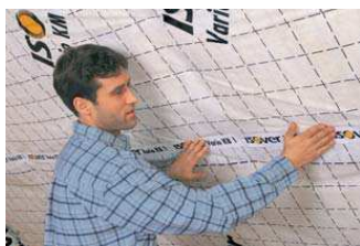
Proper installation ensures airtightness and full moisture protection of the roof construction.
