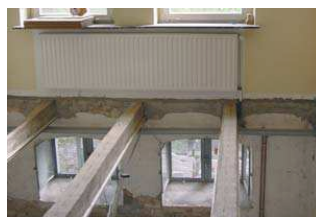
Wooden cellar ceiling, completely opened for rafter repair
