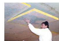
Concrete ceiling insulated from below
