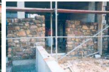
Raising the natural stone walls on the separate ring footing
