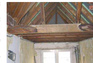
Loft ceiling opened on both sides for renovation
