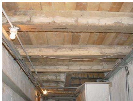
Wooden cellar ceiling, opened for insulation from below
