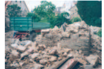
Clearing away the rubble and securing the remaining construction
