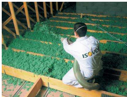
Loft ceiling opened for blowing in insulation
