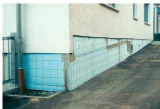
Additional insulation of outer cellar walls: only above ground (first step)
