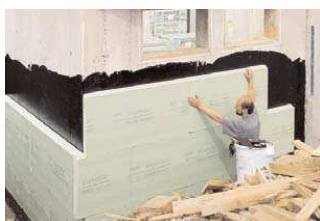
Additional insulation of outer cellar walls when replacing the waterproofing layer
