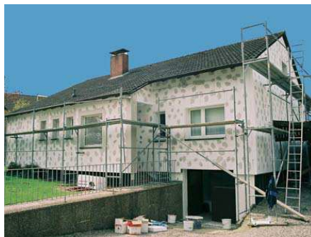
16 cm polystyrene (EPS) insulation installed from outside before the new plastering
