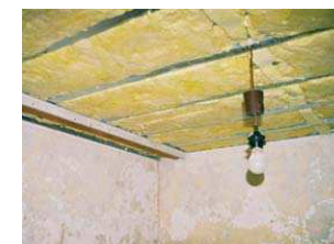
With an additional insulated metal subconstruction
