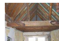
Ceiling opened from both sides
