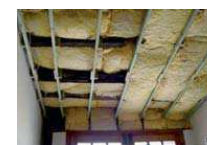
Ceiling opened and insulated from the bottom
