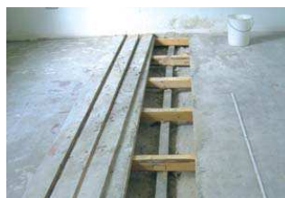
T-beam ceiling opened from the top
