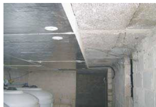
Insulation from below with 12 cm polystyrene boards
