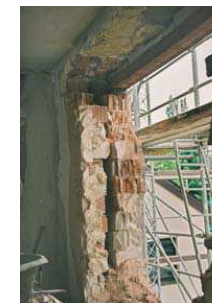
Cavity wall that has been opened around a window opening
