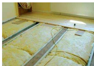
Wooden cellar ceiling with new insulation installed from the top
