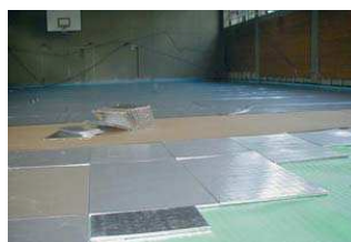
Additional sole plate insulation with vacuum panels in a sports hall (photo: Va-Q-Tec)
