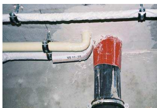
Well-sealed pipes crossing a cellar ceiling
