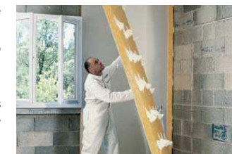
Internal insulation of an outer wall with ISOVER composite panels CALIBEL made of glass wool and gypsum board
