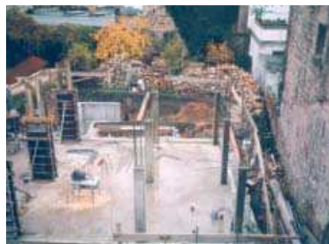
Erection of the concrete skeleton
