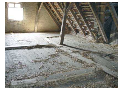
Loft ceiling only made of wooden boards – typical of old farmhouses, but now without the annually renewed straw insulation.
