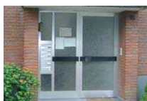
Aluminium front door of 1970 with not insulated frames
