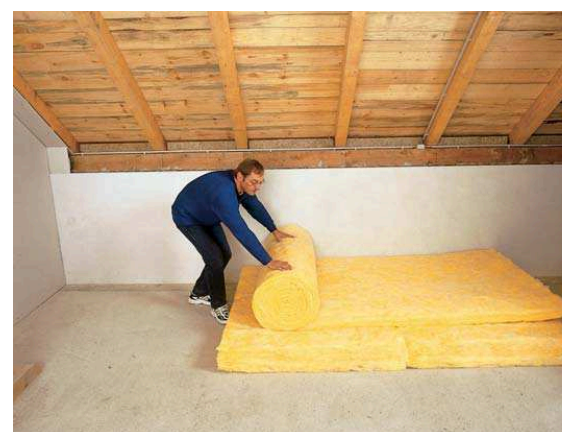
For fire protection it is important to use non-combustible mineral wool insulation.
