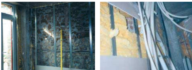
Metal frame construction facing the natural stone wall
