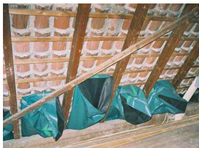
Vapour-permeable bags placed between rafters to cover later blown-in insulation
