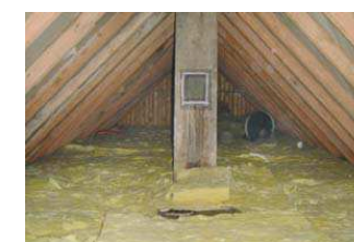
For fire protection it is important to use non-combustible mineral wool insulation.
