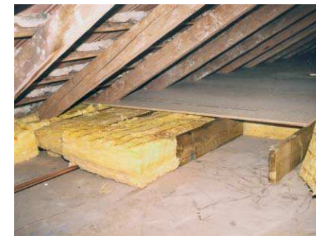
Top side mineral wool insulation and chipboard on wooden spacers
