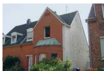
High houses: large wall areas
