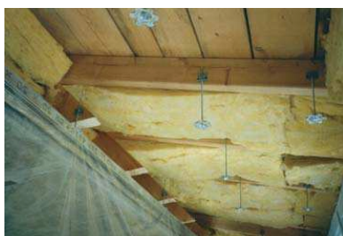
Ceiling construction of the shed dormers with ROSATWIST
