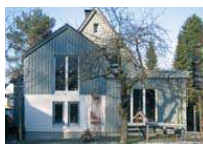
2 x 6 = 12 cm outer insulation of a solid wall with a clinker facade
