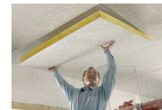
Insulation from below with 12 cm glass wool boards
