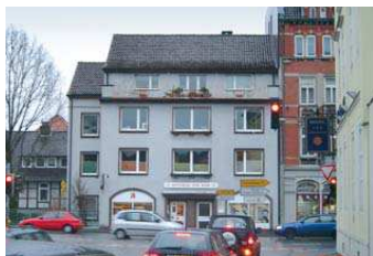
City house with bad conditions for ventilation via front windows
