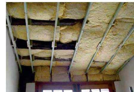
Loft ceiling insulated from the bottom: between and below the beams
