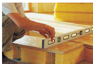
Additional sole plate insulation with ISOVER raised floor system Distansol. Special moisture and condensation protection is needed!
