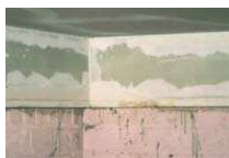
Flanking insulation of upper cellar walls to minimize thermal bridges
