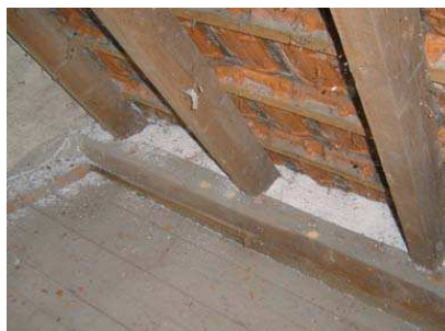
Loose granule fill between rafters made of expanded shale
