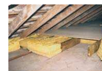
Concrete ceiling insulated on its upper side
