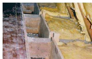
Vertical boards between the collar beams and a mineral wool filling prevent outside wind from crossing the ceiling space.
