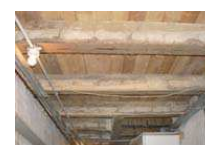
Wooden cellar ceiling opened from below
