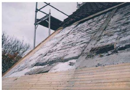
Pitched roof with lightweight stone filling, just opened from outside
