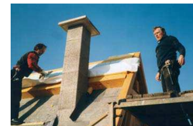
Installation of above-rafter insulation on the ridge
