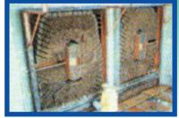
**CONDENSER:** Steam exiting the turbine is converted back into water inside the condenser as the vapor comes into contact with tubes carrying cool water from the cooling towers. Heat is transferred from the steam to circulating water which is pumped back to the cooling towers. The condensed water from the turbine is pumped back to the boiler for reuse.
