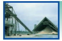
**LIMESTONE HANDLING:** Up to 12,000 tons of limestone for use in the flue gas desulfurization scrubbers is stored in a large A-frame structure. The limestone is transported by a conveyor system with a maximum capacity of 400 tons per hour. Four scrubber modules are normally operating for each unit. Each unit uses about 12 tons of limestone per hour. A spare module is available to ensure system reliability.
