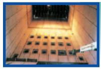
**FURNACE:** Pulverized coal is blown into the furnace where it is ignited and burned. Purified water flows through boiler tubes inside the furnace. This water is heated and becomes steam, leaving the boiler at a temperature of about 1,000 degrees Fahrenheit.
