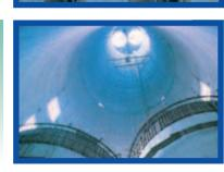
**STACK:** Flue gas leaving the scrubbers exits through the 675-foot tall stack. The outer concrete shell is constructed to protect the two inner flues from high winds. Each of the flues is made of more than one million bricks.
