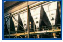
**ELECTROSTATIC PRECIPITATORS:** From the furnace, the exiting flue gas is fed into electrostatic precipitators which remove 99.7% of all fly ash produced from burning coal. Electrically charged metal plates attract the fly ash, which is deposited in large collection hoppers at the base of the precipitators. Fly ash is sent to the effluent processing area.
