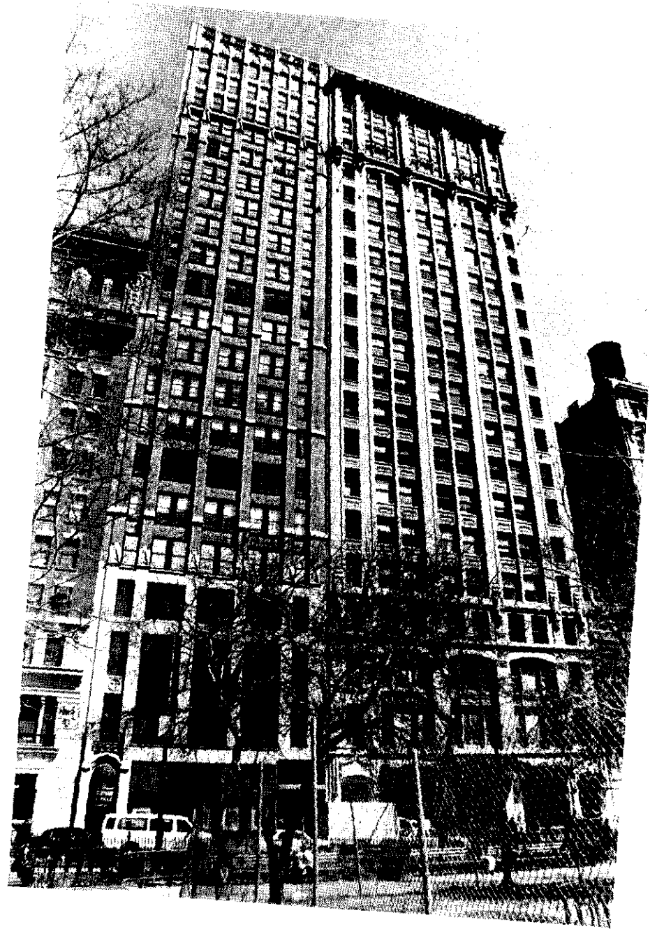
"The Goddard Building," 11-13 East 26 th Street, aka 6-8 East 27 th Street, and "The Madison Square Building," 15-19 East 26 th Street, aka 10-14 East 27 th Street. Photo: Carl Forster, 2001
