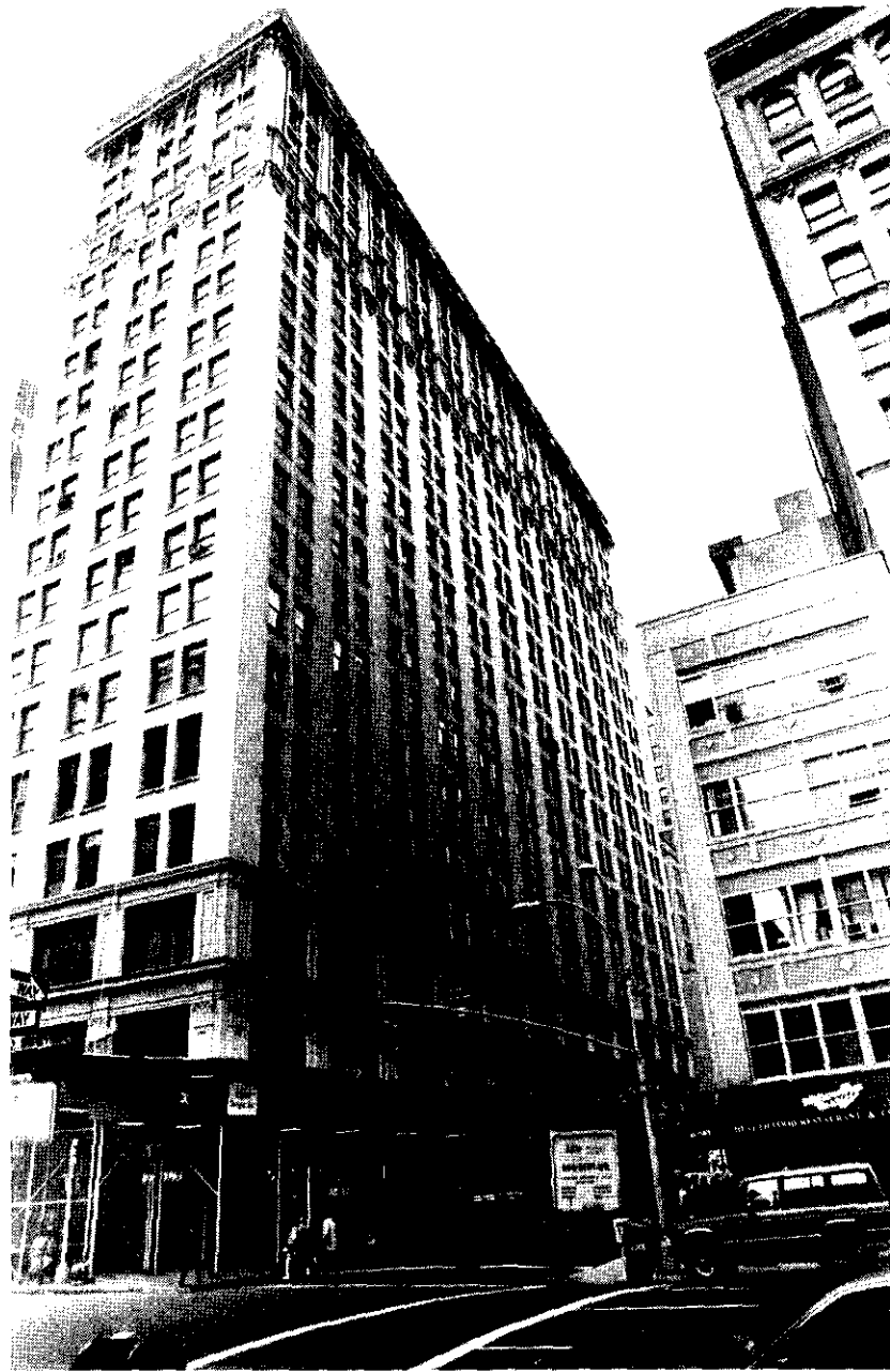
“The Victoria Building,” 228-232 Fifth Avenue, aka 2-4 West 27 th Street and 1148-1156 Broadway (Fifth Avenue and West 27 th Street facades) Photo: Carl Forster, 2001
