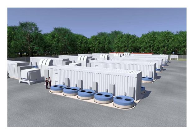
(**Above**) Artist's rendering of Beacon's 20 MW flywheel plant, as seen in close-up. The plant consists of 200 Smart Energy 25 flywheels housed below ground in concrete cylinders (blue covers seen above), along with 20 steel containers (1 per MW) placed on concrete pads. The containers house electronics and communications equipment.
